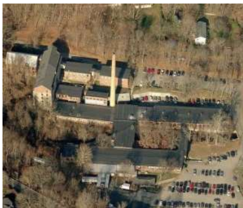
Site of Oxoboxo Lofts development
